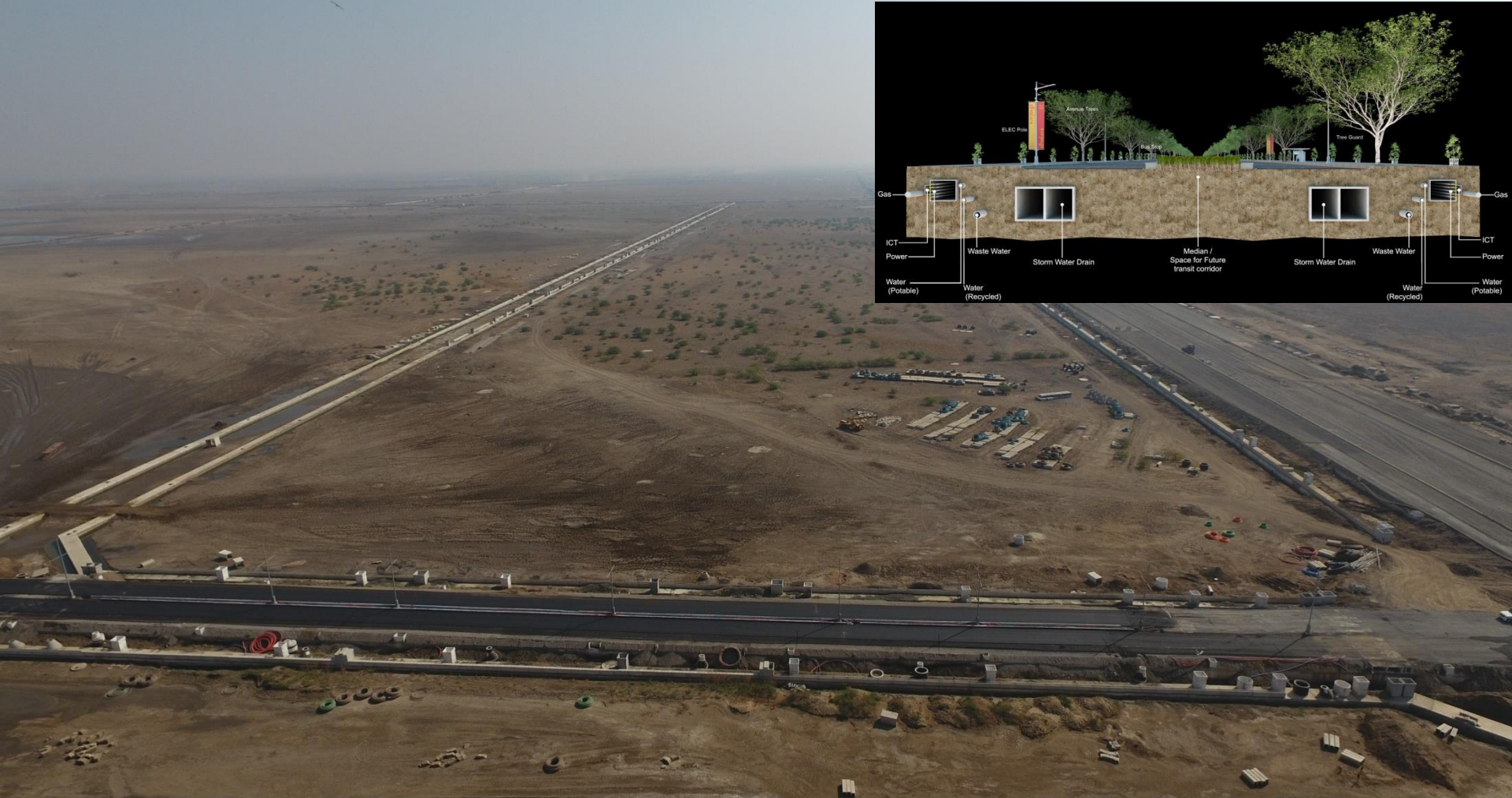
Roads & Services_B-43, E-2 & H-1 Roads
