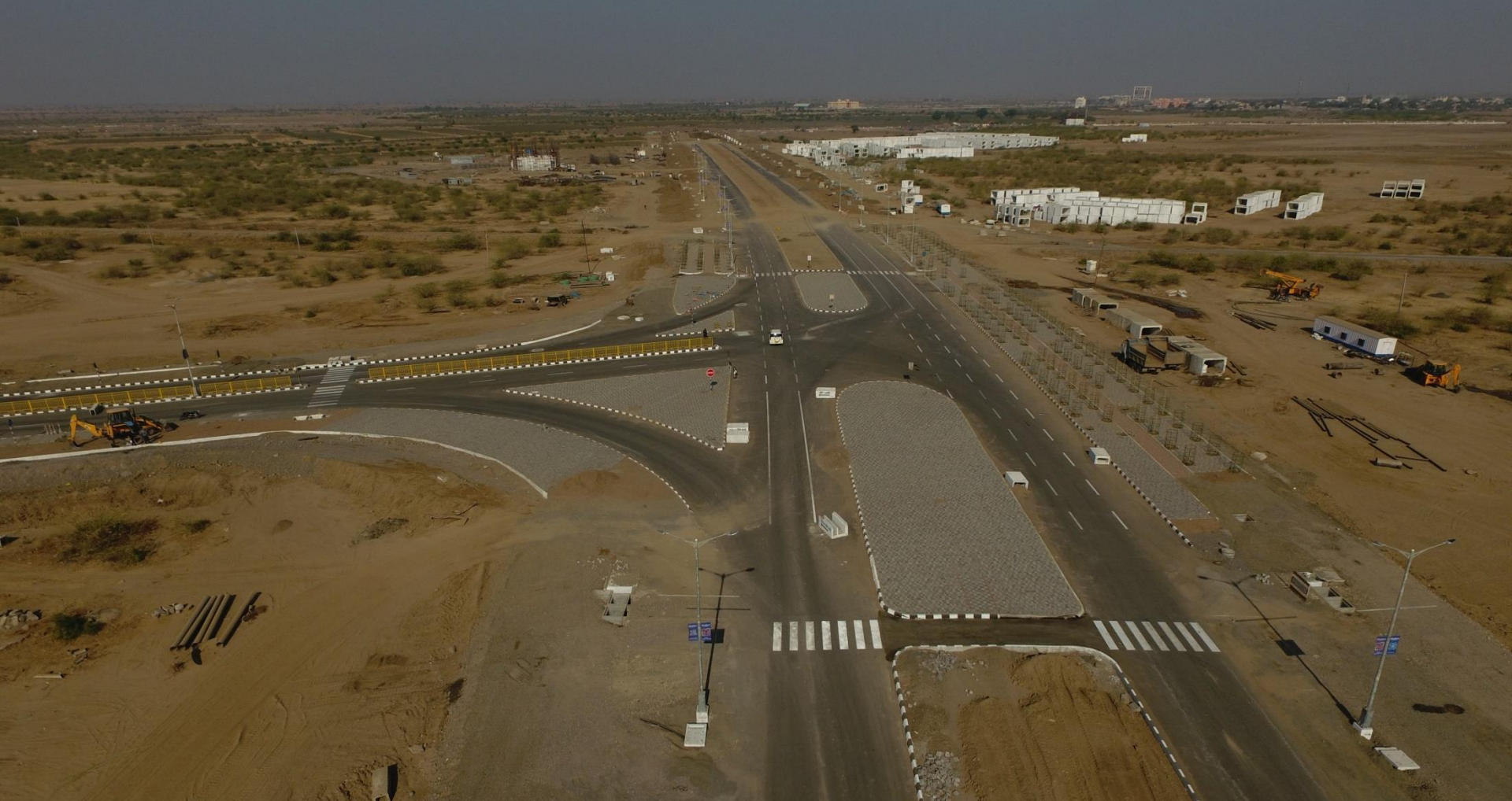
Roads & Services_G-4 & E-2 Road Junction
