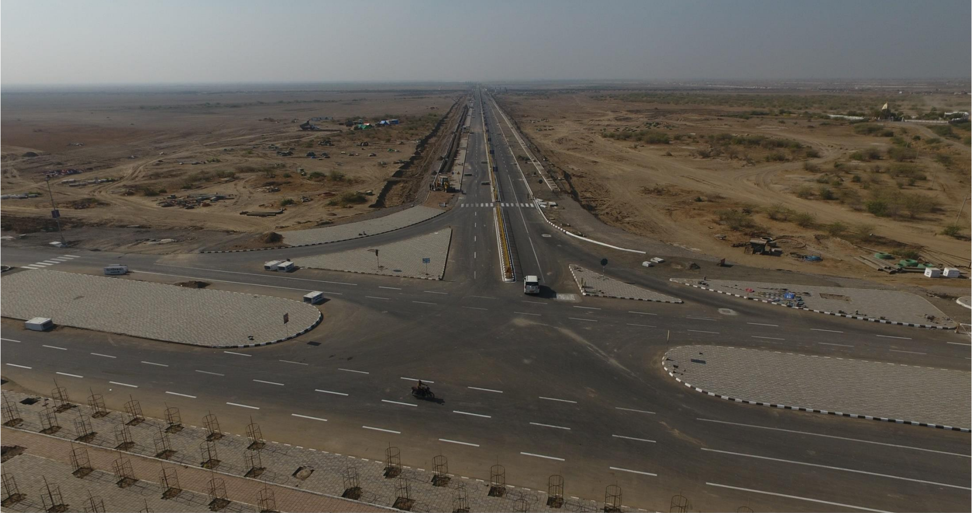
Roads & Services_G-4 & E-2 Road Junction
